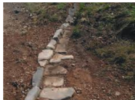
2 Creating cross drains on Blackdown to prevent erosion by rain run off
