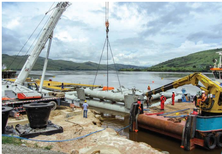
Industrial Rigging Solutions team performing heavy lift operation in Africa.
