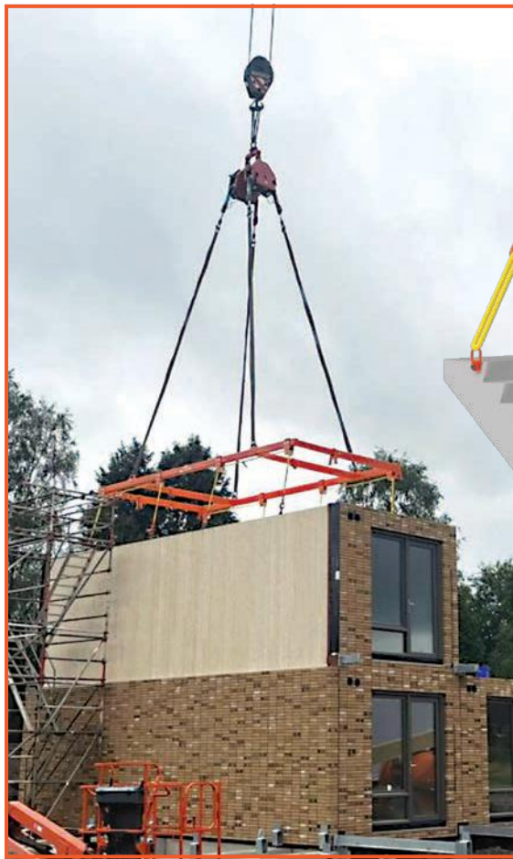
Above: The pewag Levo load balancer is frequently used to lift long, awkwardly shaped stairways. Left: The pewag Levo load balancer can be used instead of cascading spreader beam setups when headroom is limited.
