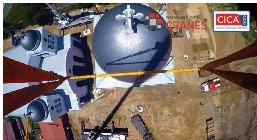
MOD Spreader Beam carefully lifting the roof dome into position.
