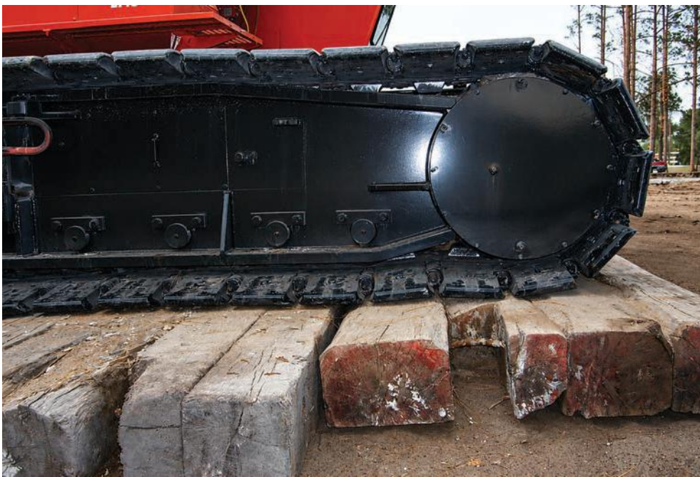
Fig. 6. Timber mats provide additional ground support necessary for sandy soils.
