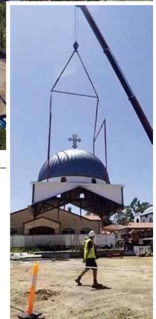
MOD 24 spreader beams in a H-pattern configuration.
