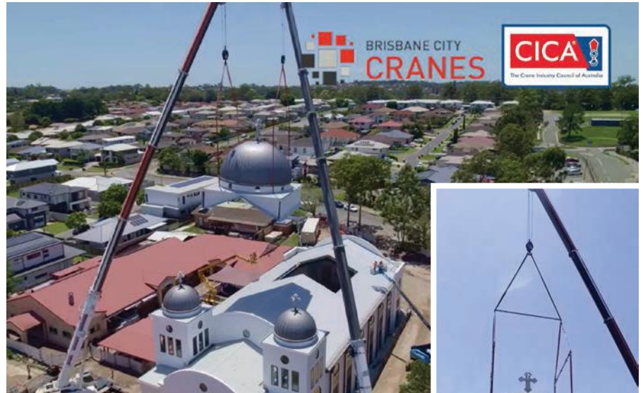
Dual Cranes relocating dome structure.
