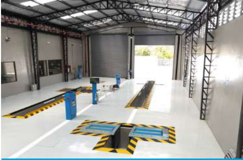
LV | HGV FULL TEST LANE
