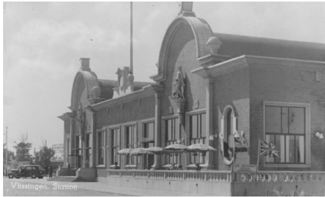
Station Vlissingen (col. DB)
