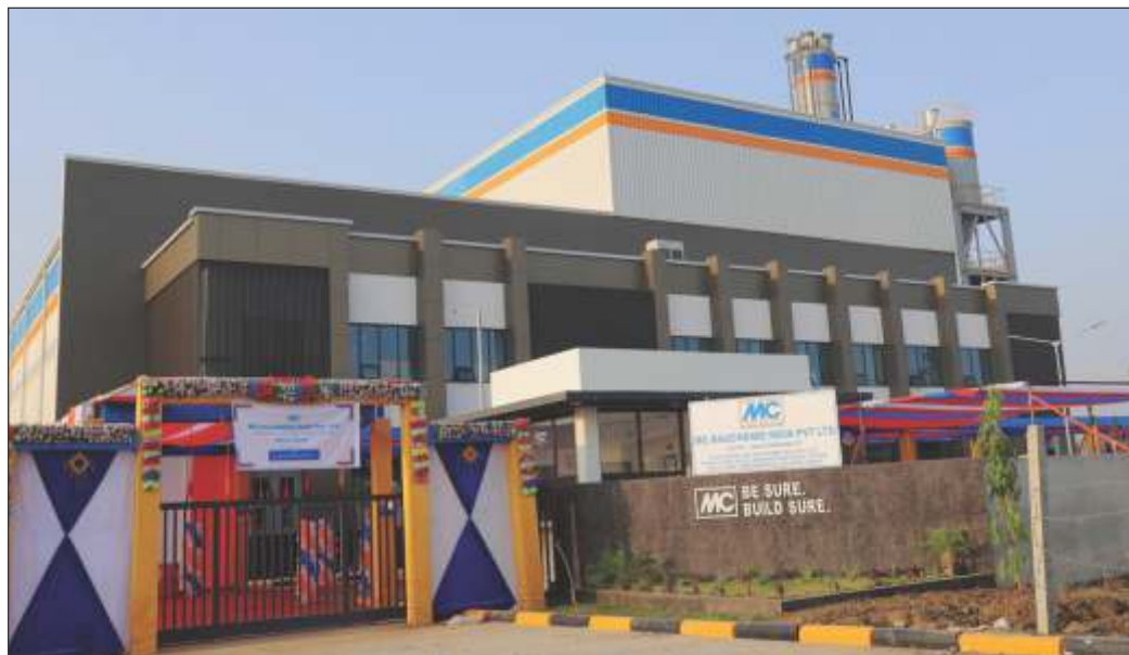
View of MC-Bauchemie India's new industrial facility in Halol.
