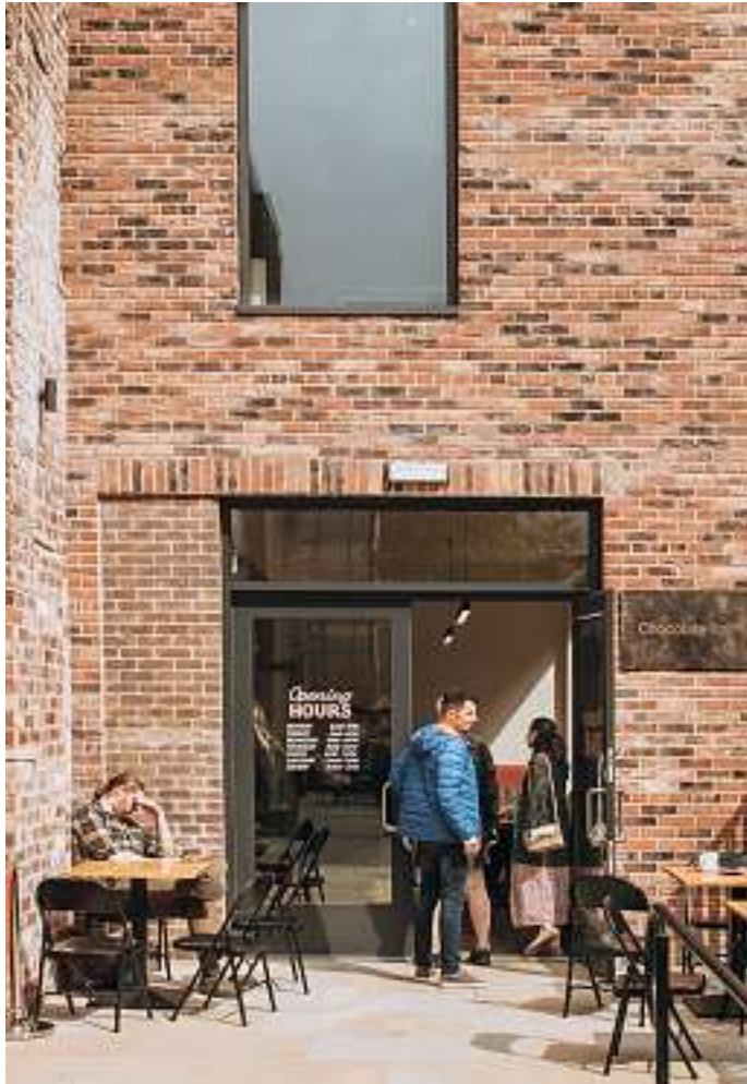
Below New windows and brickwork are carefully stitched into existing historic walls.
