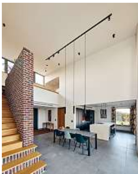
Above Concrete floors, porcelain tiles and a solid brick wall – with some characteristically sharp mortar – help with the thermal mass.
