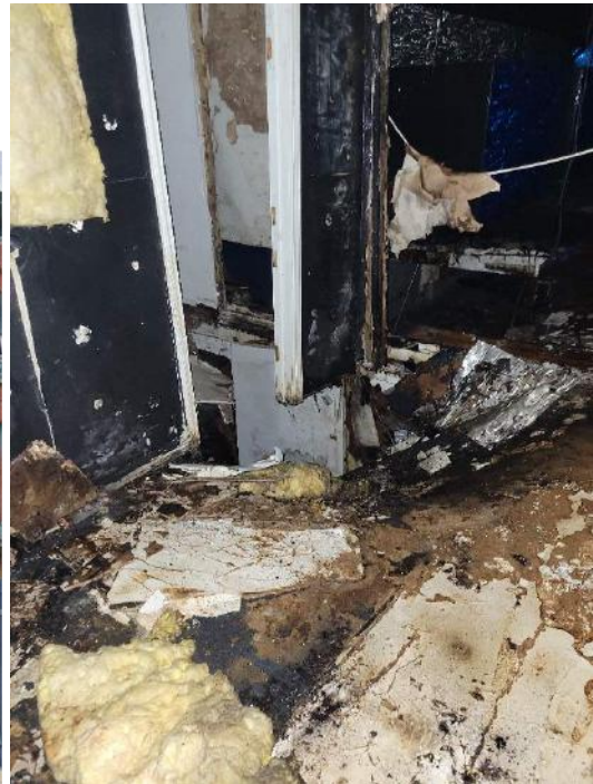
Figure 2: View of 131 N. Main front and interior floor collapse
