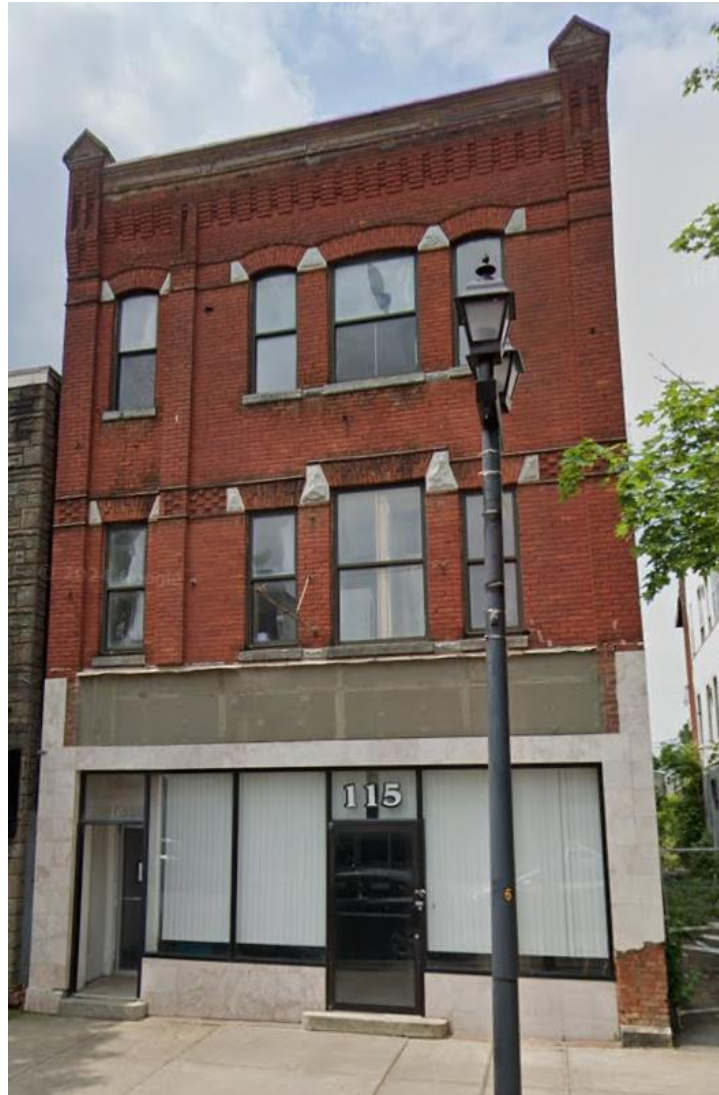
Figure 1: View of front of building
