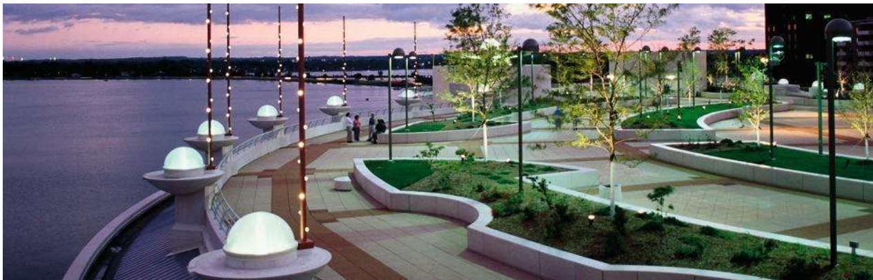
The BCP's vision, for the new improved Capital city of West End, Grand Bahama, which will serve as the location for the Office of the Prime Minister on Grand Bahama Island.
