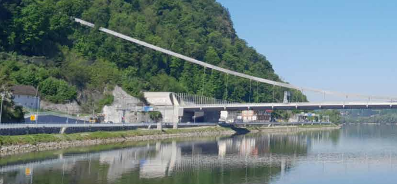
A true suspension bridge: the 500-metre-long suspension cables of the Danube bridge in Linz are anchored in the rock.
