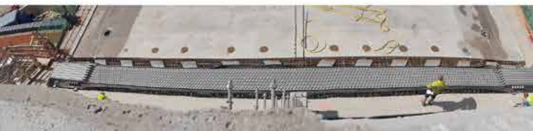
Expansion joint construction at the tunnel entrance. The image clearly shows the rhomboid plates welded on for noise reduction.
