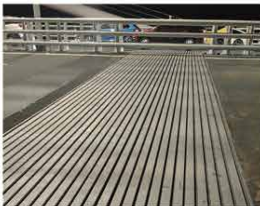
Left: The expansion joint in place ready to be encased in concrete. The boxes containing the swivel joists are visible on the left.
