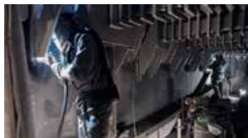
The new MSM® swivel joists are welded onto the steel bridge over the Rhine. Photo: Andreas Hantschke
