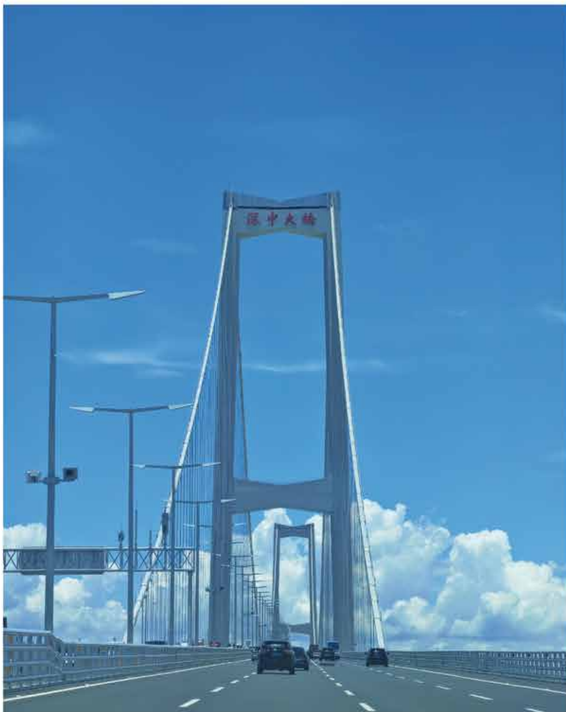
The main bridge of the Shenzhong Link, with its 1,666 m main span and bridge deck 91 m above the sea.
