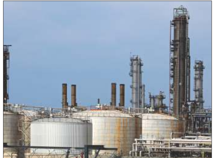
Axis Solutions Pvt Ltd serves a diverse range of sectors including oil & gas, petrochemicals, refineries, power plants, coal and mining, and chemicals.
