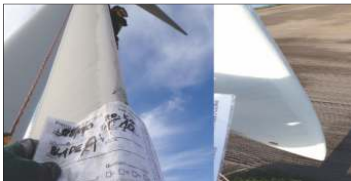
Leading edge repaired and protected with Belzona 5711 and Belzona 5721.
