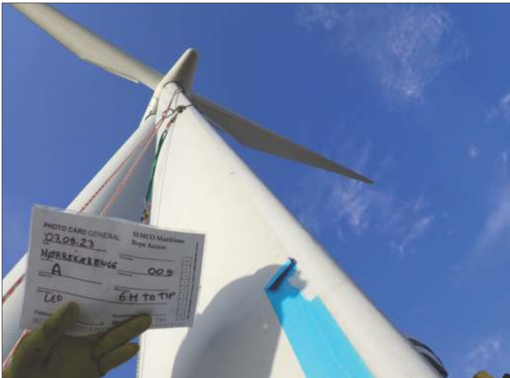
Leading edge protection of wind turbine blade using polymeric technology.
