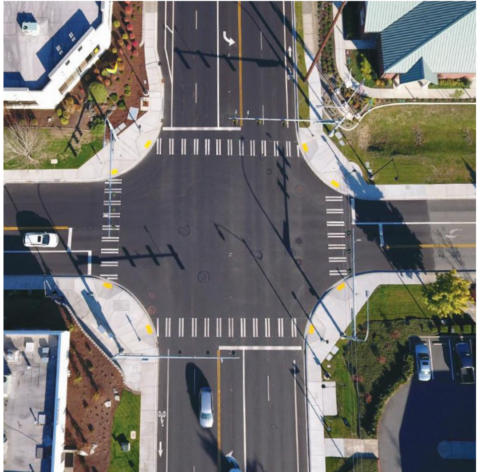
NW Bucklin Hill Road and Mickelberry Road
