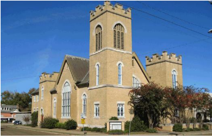
FUMC Yazoo City; Moorish Revival Port Gibson
