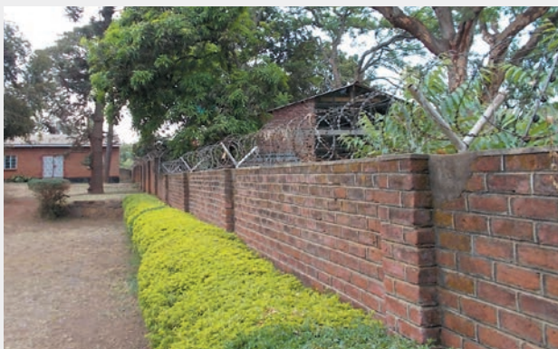
A wall between a liaison office for JICA volunteers and a neighboring house, topped with barbed wire to deter intrusion. (The photo was taken by a security advisory mission dispatched to the country.)
