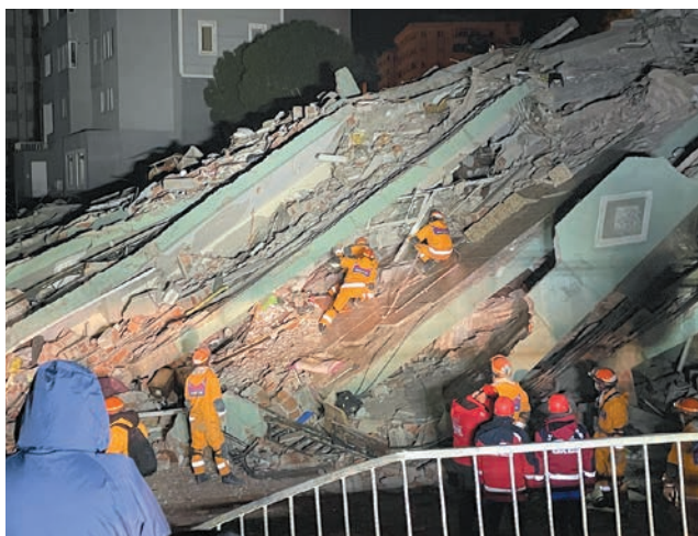
Turkey: The JDR Rescue Team conducted search and rescue operations while local residents looked on. The teams worked for seven days from the day after the quake hit.
