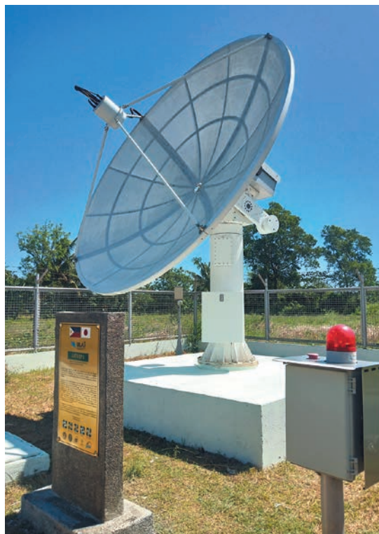
Philippines: An antenna for a local user terminal (a ground satellite data receiving station) provided under the Project for Development of Extreme Weather Monitoring and Information Sharing System. With the use of satellite data thus received, the project developed a system to forecast extreme weather events.
