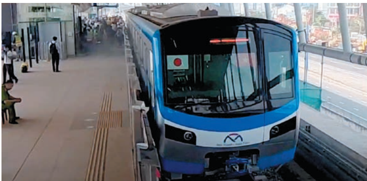
Viet Nam: A ceremony for the launch of a test run in the Ho Chi Minh City Urban Railway Construction Project (Ben Thanh–Suoi Tien Section (Line 1)) in December 2022. With Japan's development cooperation, Viet Nam is constructing an urban railway that includes the country's first underground section. The railway is expected to take root as a popular means of transportation.
