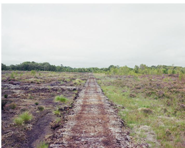
Bunding used for bog restoration, Timahoe South, County Kildare, 2024.
