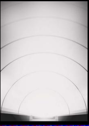
Typical light spill from flood light
