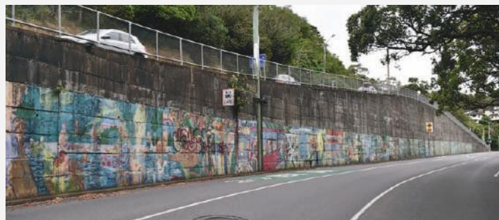
The Chaytor Street retaining wall. Photo: Frank Neill.
