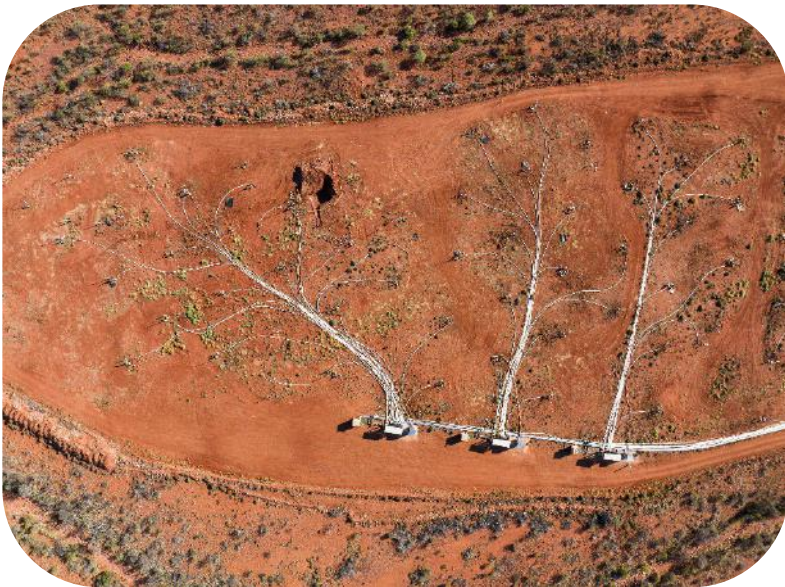
Well network and pipework at Beverley
