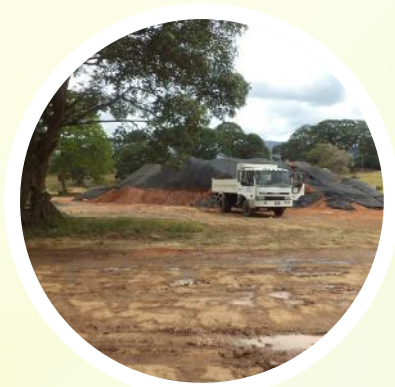
Stockpiles located within designated areas and protected by geo-textiles
