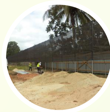
Installation of dust screens and hoarding along site perimeter
