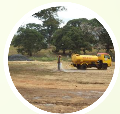
Regular application of water to reduce dust emissions.
