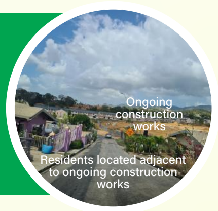
Figure 2: Ongoing construction works at housing development site.
