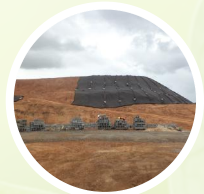
Geotextiles protecting exposed slope
