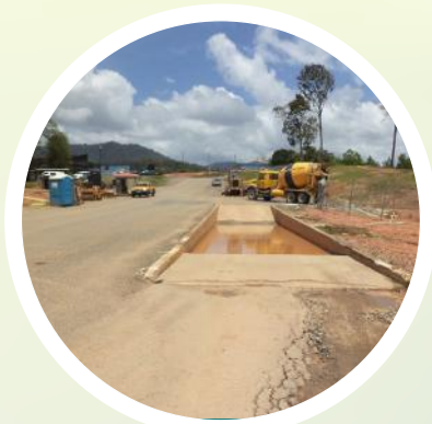
Washbay established for vehicles entering and exiting construction site
