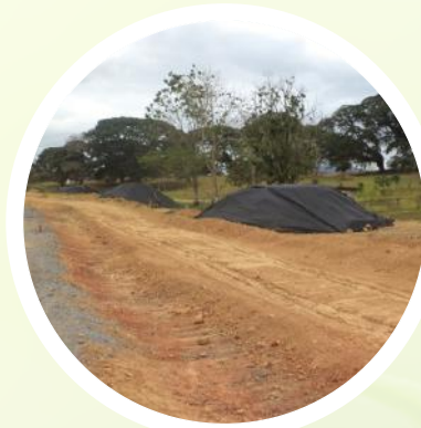
Stockpiles located within designated areas and protected by geo-textiles
