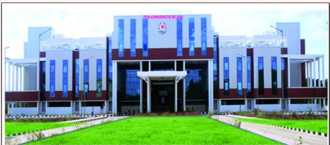
JNTUA ADMINISTRATIVE BUILDING, ANANTHAPURAMU
