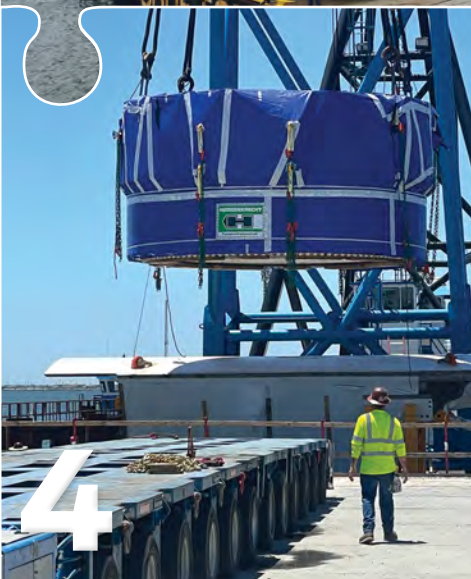
1 An aerial view of the assembled tailskin. 2 Pieces of the shield are moved from the barge to the island. 3 Crews assemble the cutterhead. 4 A crane lifts the main drive. 5 Inside view of crews welding together the tailskin.
