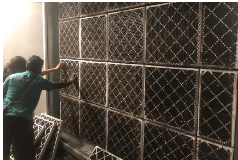
CONTINEWM®, a patented ceramic net which acts as an infrared emitting filter from Japan that is testbedded at LogisTech in Singapore.
