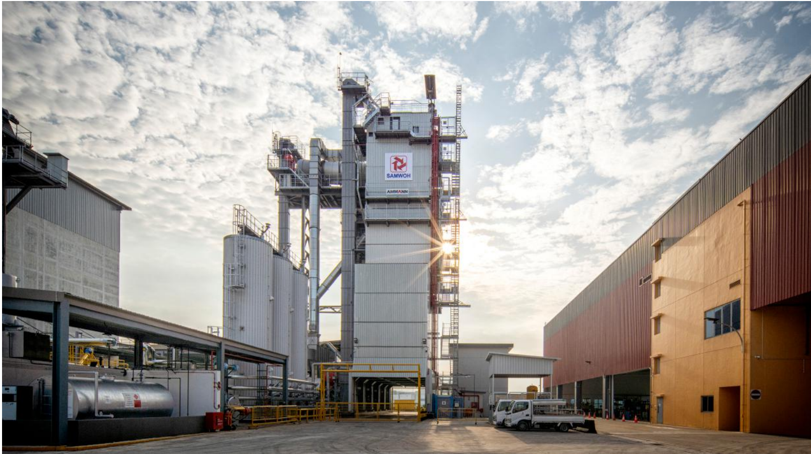
Samwoh's newest asphalt production plant is 15 percent more energy efficient than conventional plants and can achieve a carbon abatement of 1,220 tonnes per year.
