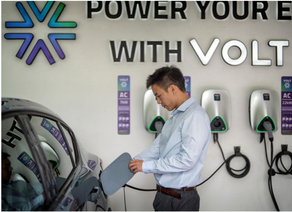
Keppel Volt electric vehicle chargers are available at Keppel Infrastructure @ Changi.
