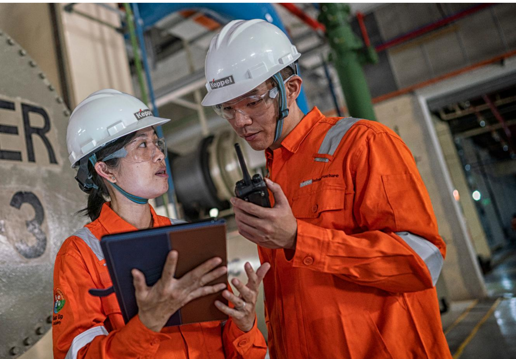
Keppel Infrastructure @ Changi is annexed to Keppel DHCS's Changi District Cooling Systems Plant.
