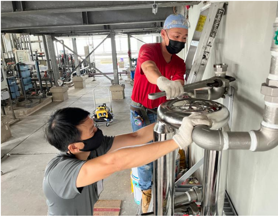
A water treatment solution for cooling towers from Singapore that is being testbedded at CapitaGreen in Singapore.
