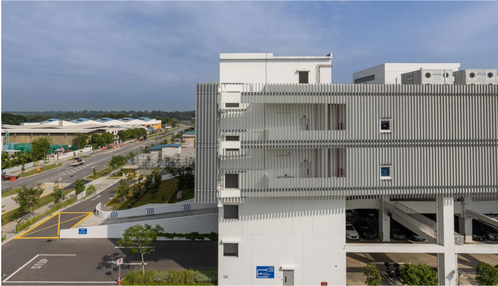
The double fins cladding on the East and West of the building diffuses direct heat and allow for a cooler interior.
