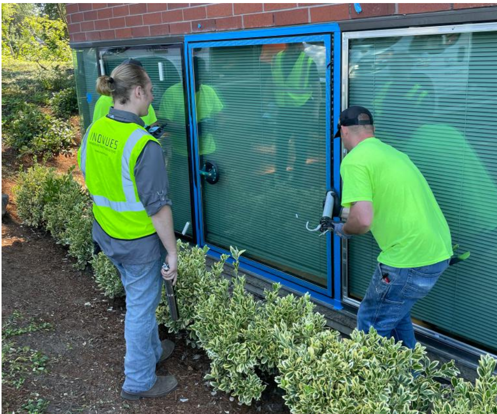
An insulating glass retrofit technology from USA that is being testbedded at the first level of Creekside 5 in Portland, Oregon.
