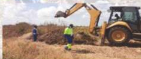
Water Pipe Trenching
