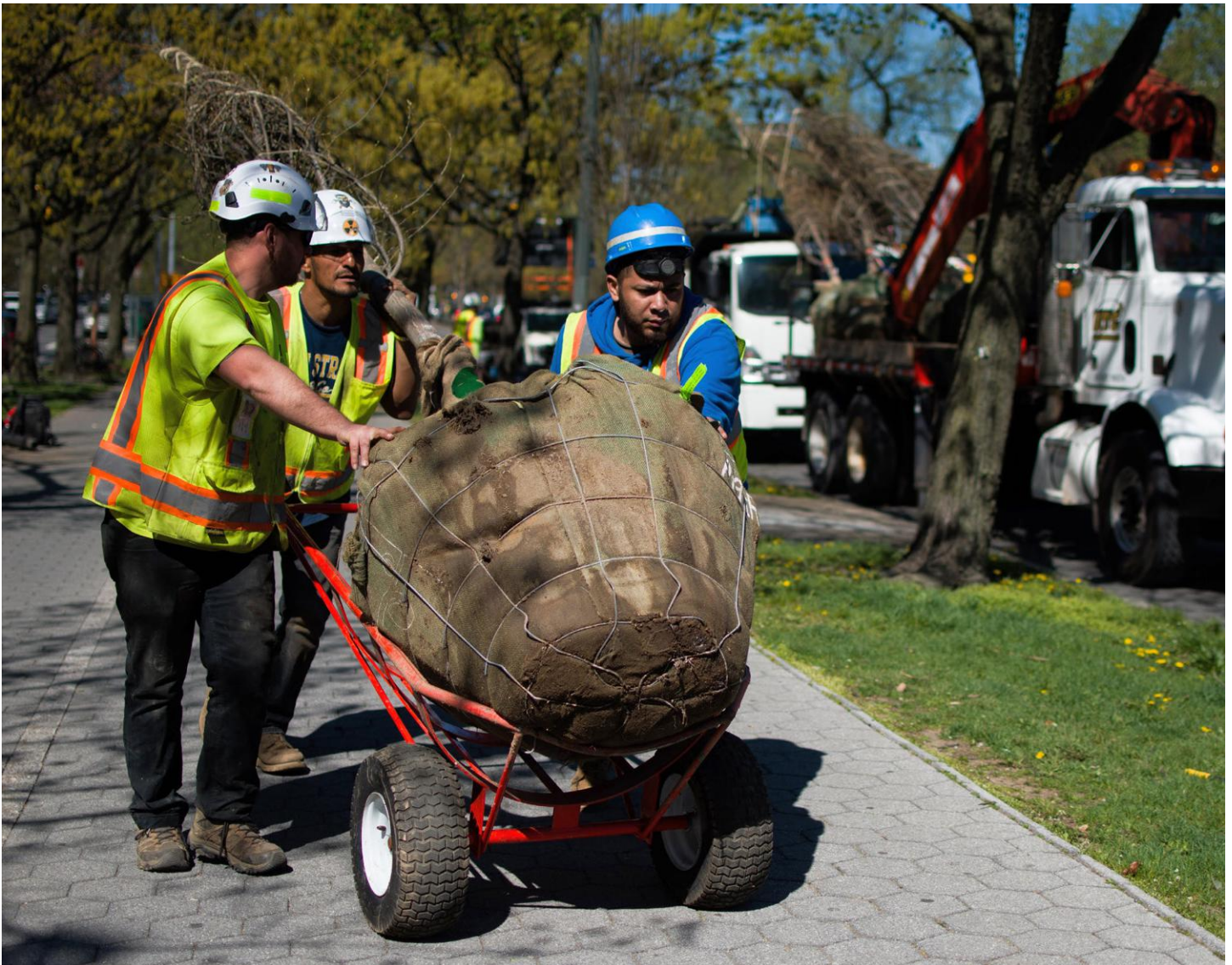
Contractors move large B&B stock toward a park planting site.
