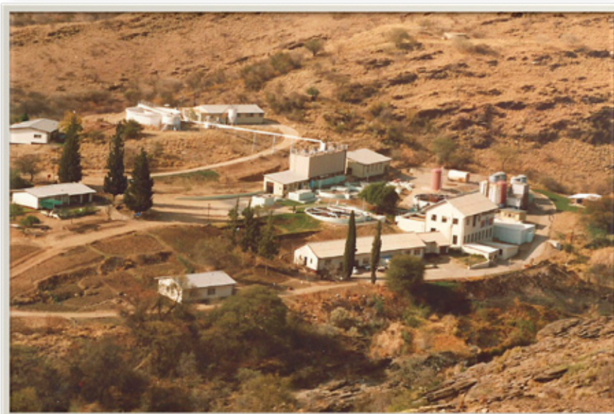
1976 – 1980 Goreangab Mark II, high lime treatment and ammonia stripping, 4.8 Ml/d
