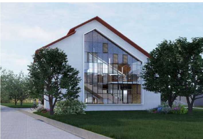
Louvre windows to allow natural cross ventilation, allowing wind to pass through and maintain thermal comfort naturally.
