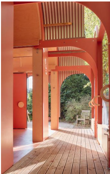
THE BLOOMING SHED, ENFIELD BETWEEN ART AND TECHNOLOGY (BAT) STUDIO FOR NORTH LONDON NHS FOUNDATION TRUST VALUE: £40,000 GIA: 30M 2 PER M 2 : £1,356
