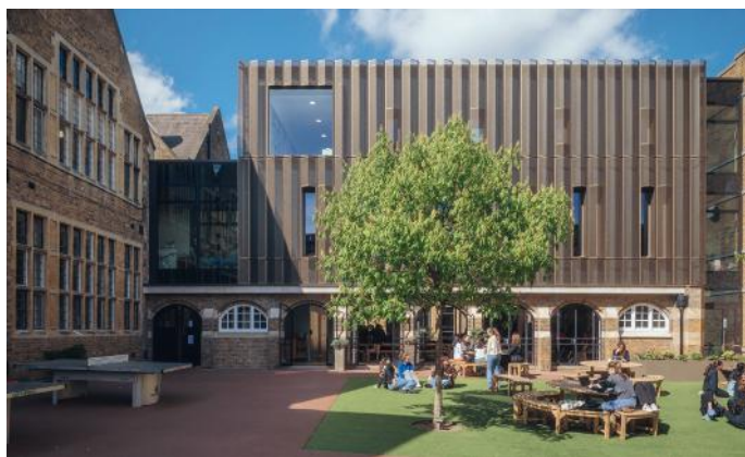
GODOLPHIN AND LATYMER SCHOOL, HAMMERSMITH & FULHAM WALTERS & COHEN ARCHITECTS FOR GODOLPHIN AND LATYMER SCHOOL VALUE: CONFIDENTIAL GIA: 1,193M 2
