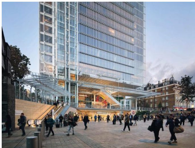
PADDINGTON SQUARE, WESTMINSTER RENZO PIANO BUILDING WORKSHOP (PARIS) IN COLLABORATION WITH ADAMSON ASSOCIATES (LONDON) FOR SELLAR VALUE: CONFIDENTIAL GIA: 63, 617M 2
