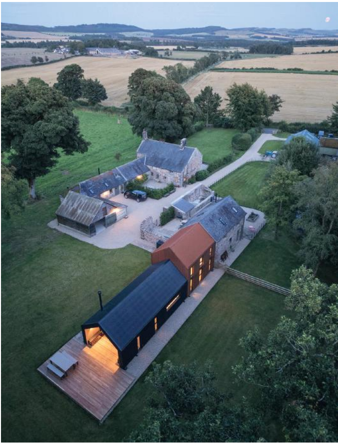
THE LIMEWORKS, NORTHUMBERLAND STUDIO-NORTH FOR JAMES AND KATIE KEMP VALUE: £378,500 GIA: 167M 2 PER M 2 : £2,266
