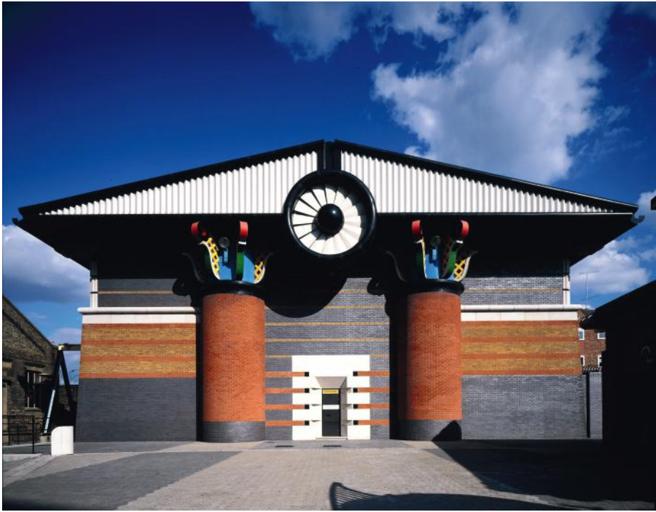
Above: The 1988 London pumping station designed by John Outram was a po-mo Award-winner.
