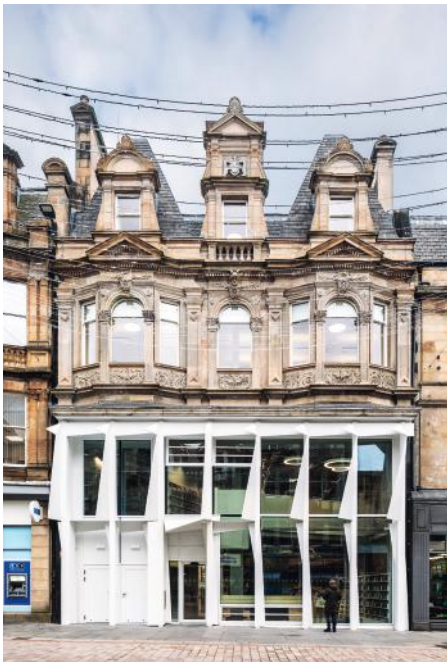
PAISLEY CENTRAL LIBRARY, PAISLEY COLLECTIVE ARCHITECTURE FOR RENFREWSHIRE COUNCIL VALUE: £4.2M GIA: 1,075M 2 PER M 2 : £3,907
