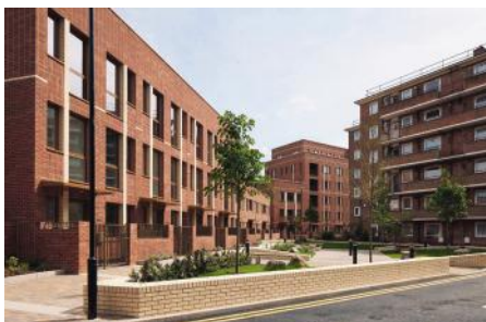
ROWAN COURT, HARINGEY SATISH JASSAL ARCHITECTS FOR HARINGEY COUNCIL VALUE: CONFIDENTIAL GIA: 4,576M 2
