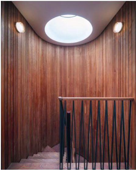
Left: Cherry slats now line the internally insulated stair tower. The circular rooflight is an original one.
