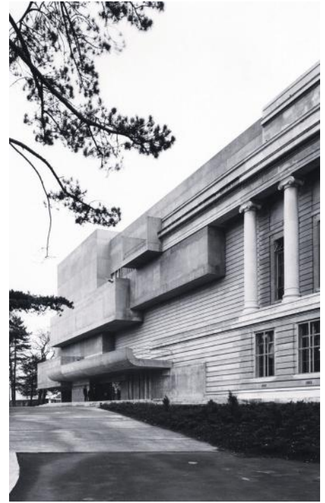
Above: Francis Pym's classically inflected concrete extension to Ulster Museum was a 1972 winner.
