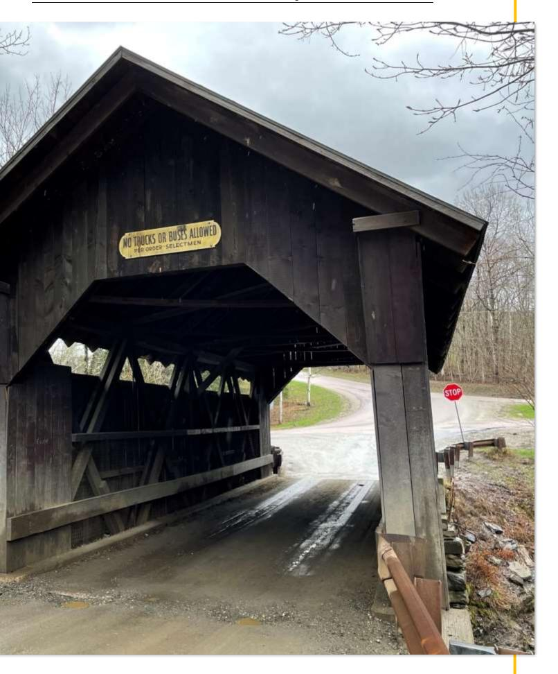
easy to build. It was also innovative because of it used vertical iron rods. The rods were secured with bolts between the diagonal beam and if the joints loosened, the bolts could be tightened. This design solved a major problem with bridges made entirely of wood.
