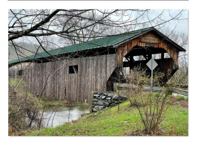
protected the bridges themselves. Exposure to harsh weather elements can lessen the life of a bridge, however, if covered, it can last a century or more. Sides and roofs made the structures more durable. Sides, in particular, helped farmers get their cattle over the bridge, as the sight of rushing water made them balk.
