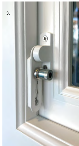
Photo No. 3 – Casement restrictor
