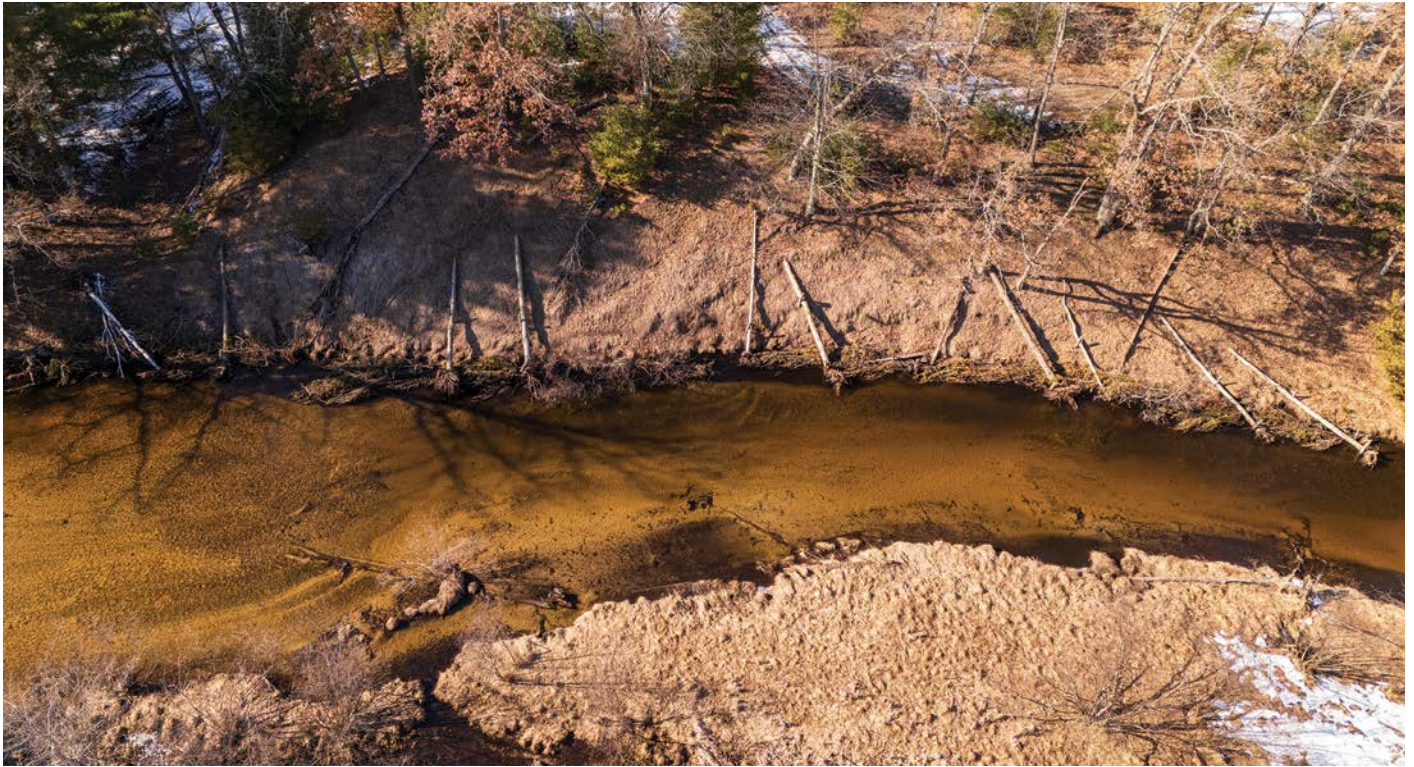
Several trees and rootwads now line the eroding bank along this river section, providing habitat and stabilizing the streambank.
