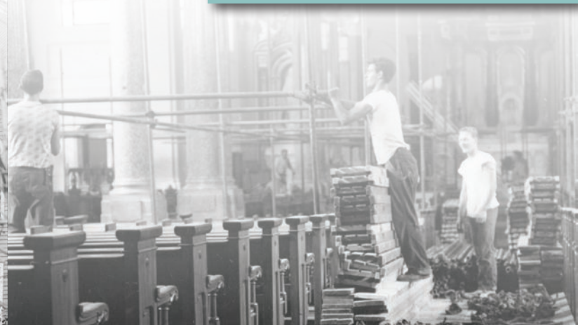
Renovating Sacred Heart Chapel
