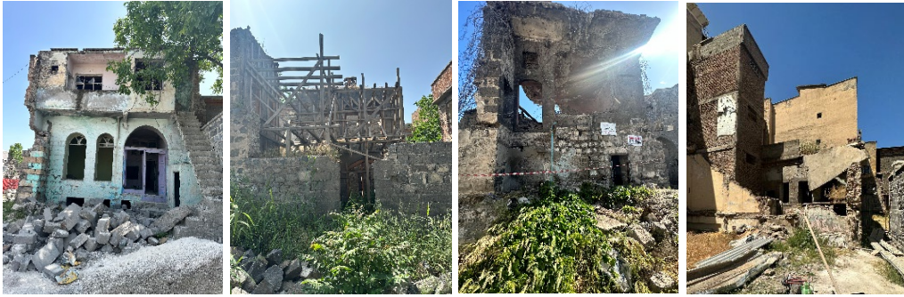
Figure 3: Severely damaged buildings
