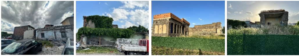
Figure 4: Buildings with minor and moderate damage
