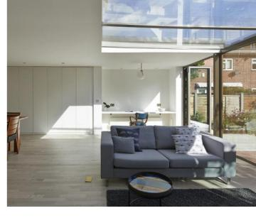
The new rear elevation contains a central fixed glazed panel that is seemingly wrapping up and over to become a skylight. The architect used uncoated brass Microlouvre Koolshade® fabric laminated into the glass as a means of solar gain control, enabling views whilst reflecting sunlight. The customer also specified that the solution must also allow for natural daylight and views out to be maintained.
