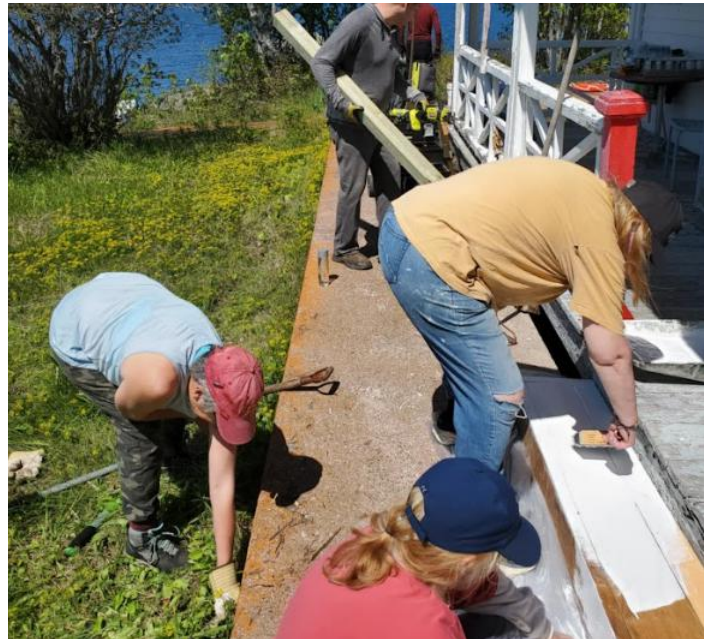
Canadian Lighthouses of Lake Superior: Volunteers cleaning around the keepers dwelling, re-painting parts of the fog alarm building, and pouring concrete for a new pay station box. Over 100 volunteer hours were completed on this day! Photograph from Paul Morralee.
