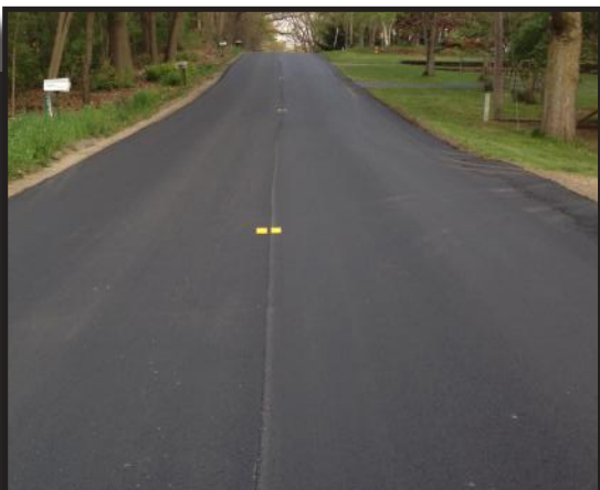
HMA paving on JK Avenue
