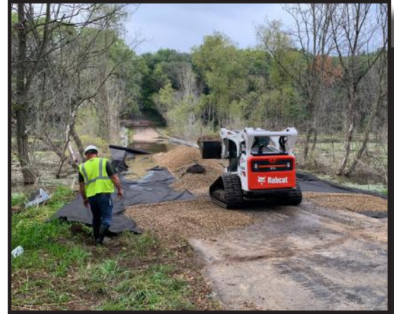
Aggregate lift on 8th Street bridge
