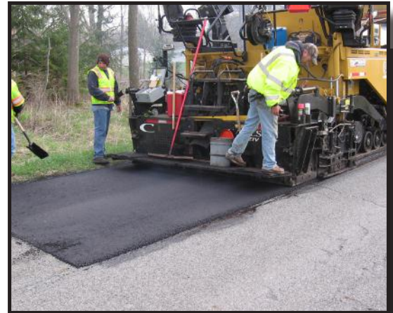
HMA wedge on V Avenue
