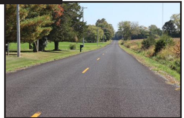
Chip seal trial on V Avenue
