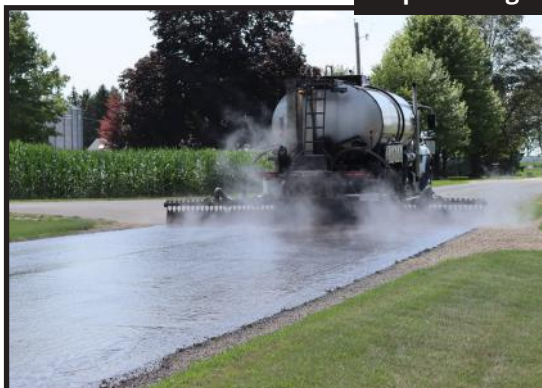
Chip seal/fog seal on VW Avenue
