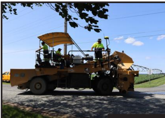
Chip seal/fog seal on VW Avenue
