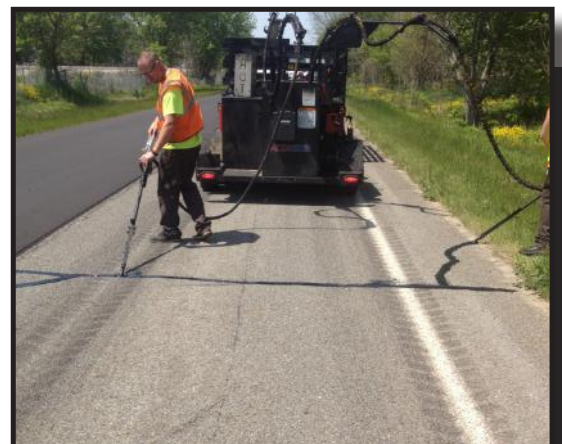
Crack fill on K Avenue
