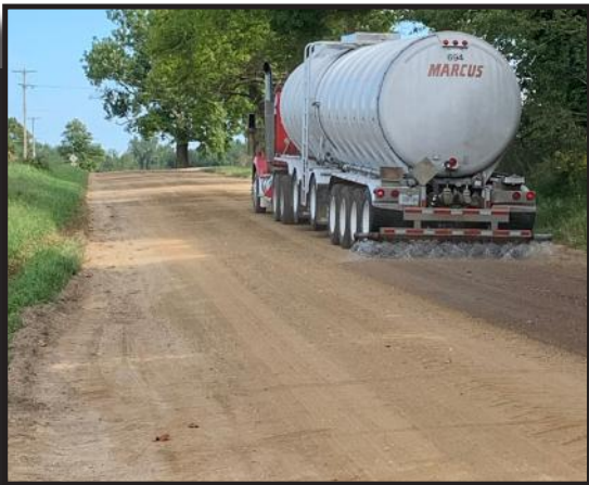
Applying dust control on 40th Street
