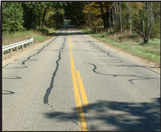
Crack seal on O Avenue
