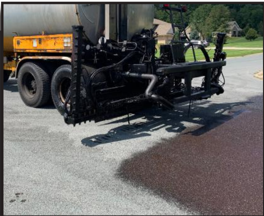
Fog seal in Oshtemo Township
