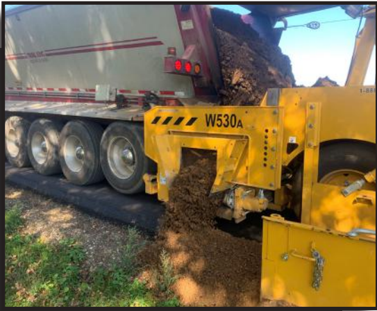
Placing shoulder gravel on XY Avenue
