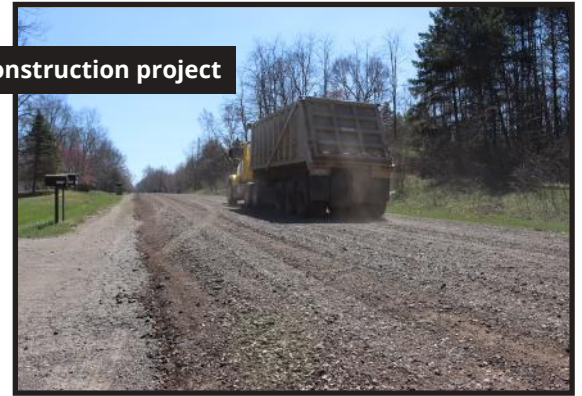
Chip seal/fog seal on AB Avenue
