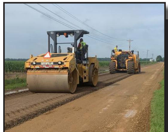
Pulverizing XY Avenue
