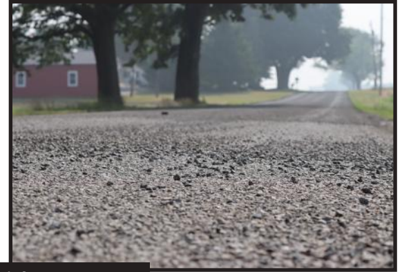
Chip seal trial on V Avenue
