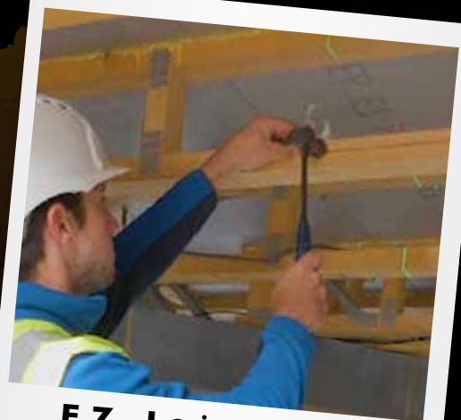
EZ Joist Clip Attach Side-on
