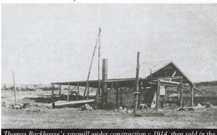
Thomas Backhouse's sawmill under construction c.1914, then sold in the early 1920s to Junction North Broken Hill Mine Ltd.
