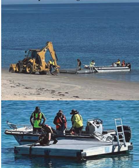
The pontoon being re-installed
