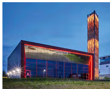
A look inside Queens Quay's water source district heat pump system
