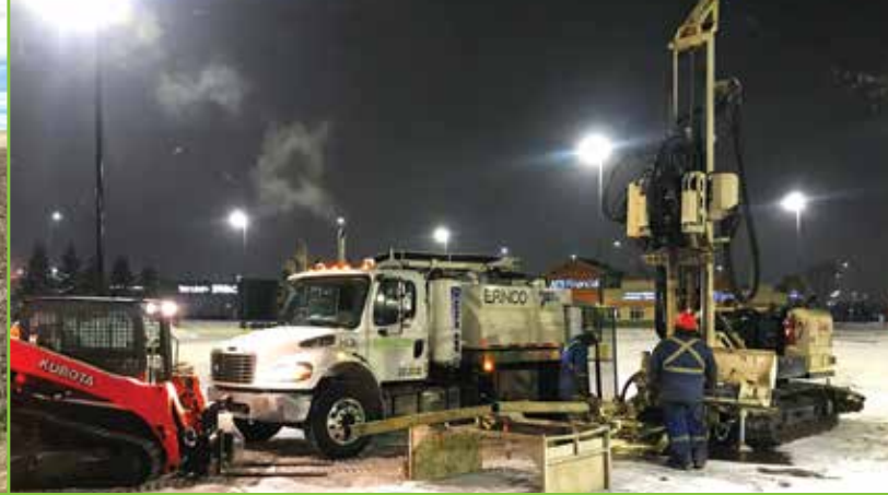
• PHASE 2: LOCATING, DRILLING, HYDROVACUING, TEST-PITTING, SNOW CLEARING, RIG MATS, SLASHING, MULCHING
