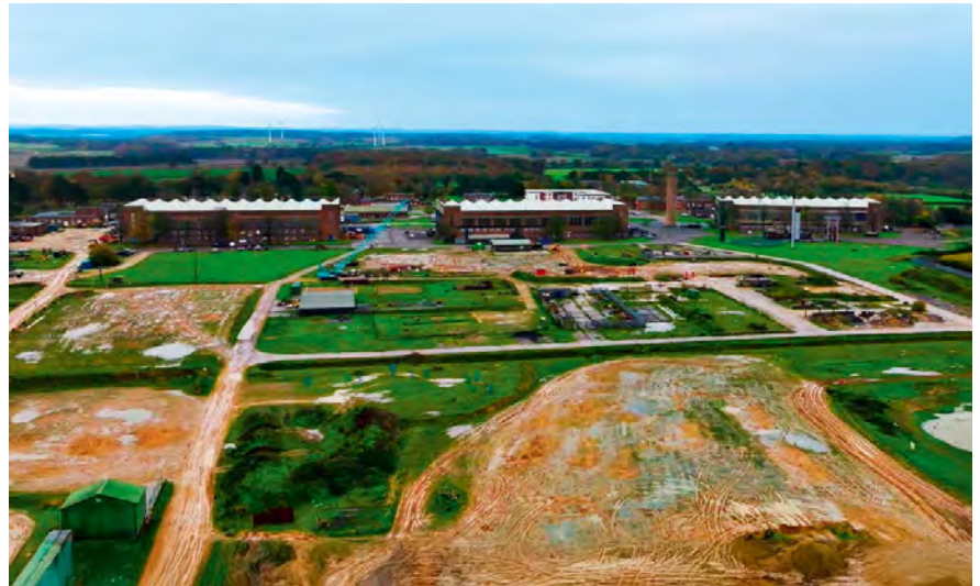
NCC extensive land reflecting a real-life construction site
