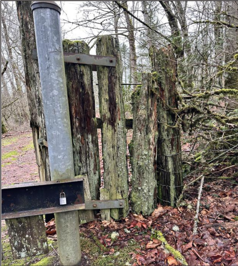
Part of Existing Gate (Right / East Side)
