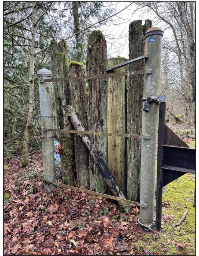
Part of Existing Gate (Left / West Side)
