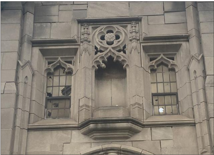
FIGURE 33: Salvageable Stone from City Methodist Church Much of the limestone from City Methodist Church is in reusable condition, and some is exquisitely carved. The tracery saved from this deconstruction process could be sold, generating income for the city.
