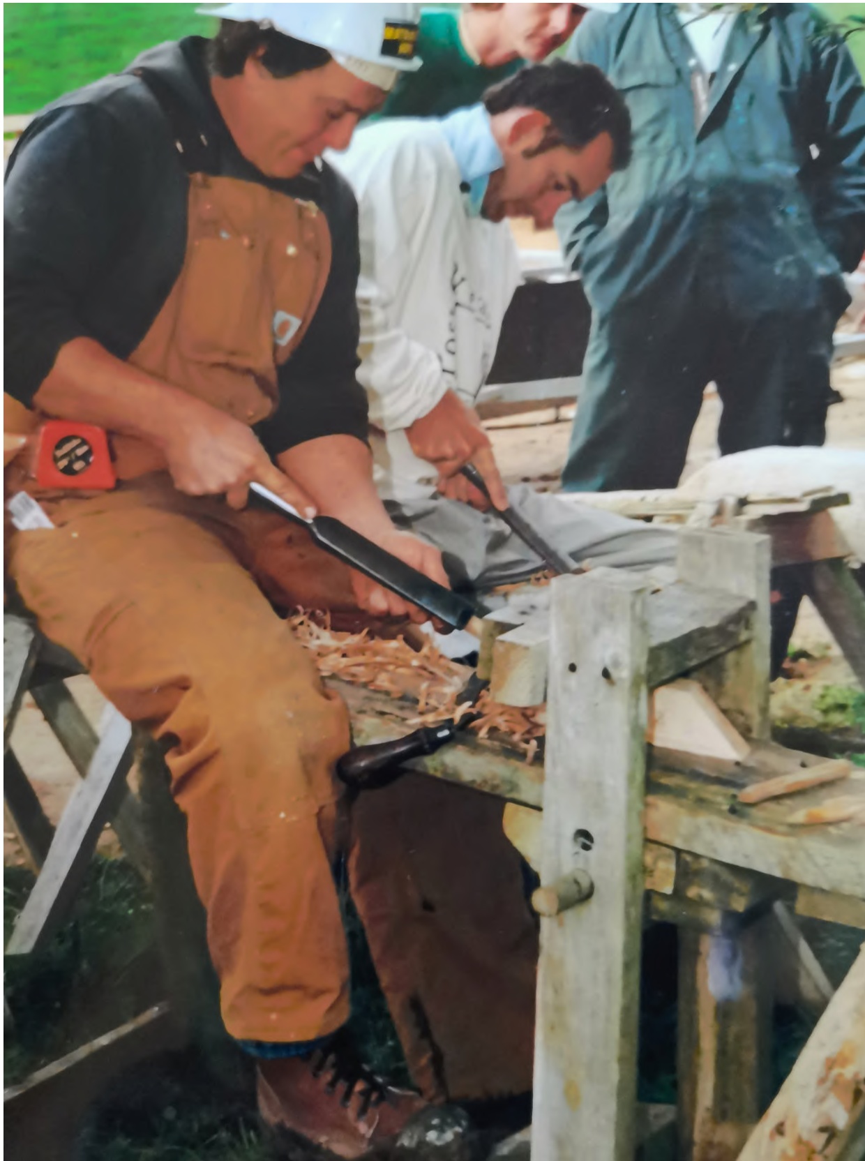
Making pegs in a team. Some 400 would have gone into the frame to secure the joints.
