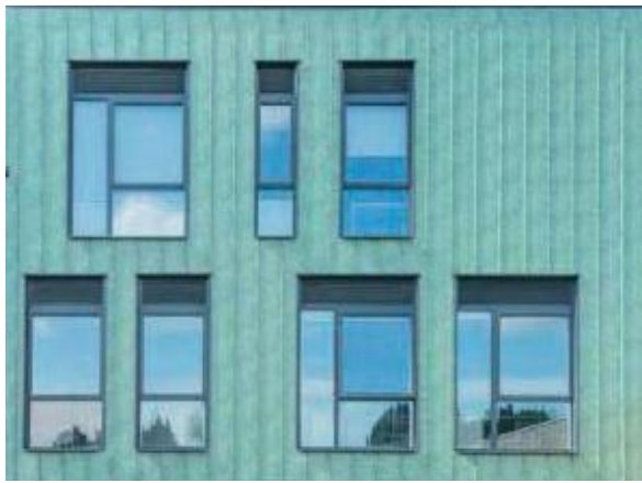
Aluminium Standing Seam Cladding System - Copper patina effect finish
