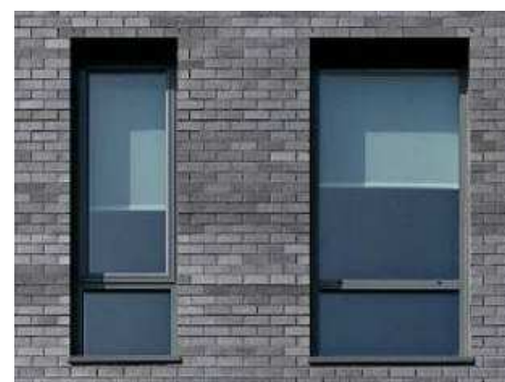
Window and Curtain walling - PPC Aluminium Frames - Dark Grey
