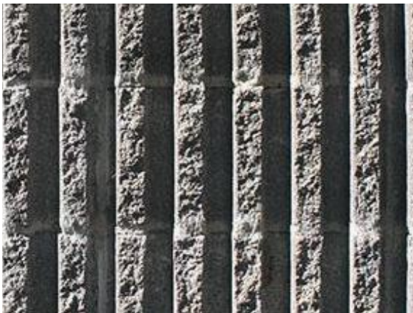
Facing concrete split face blockwork - Grey
