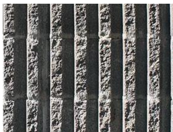
Facing concrete split face blockwork - Grey
