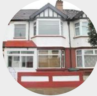
Sovereign House Tottenham Hale, London N17 London Borough of Haringey 5 person, mixed occupancy 16/17yo
