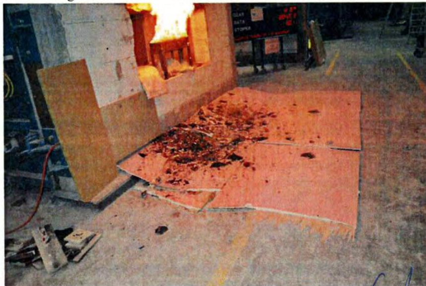
Fig. 40. View of elements which fell off during the test – the weighed elements on the left
