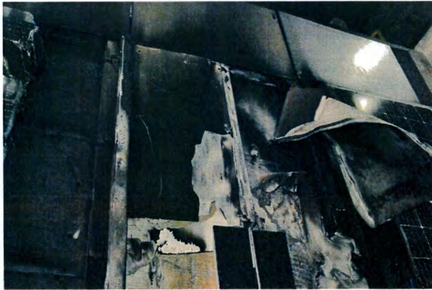
Fig. 44. View of the test element after the test - details
