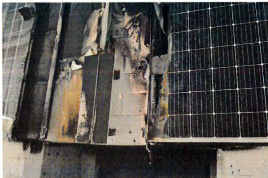
Fig. 46. View of the test element after the test - details
