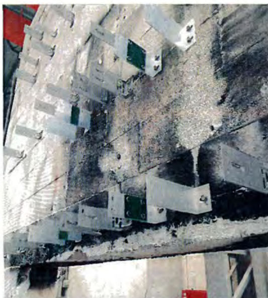
Fig. 5. View of the brackets applied
