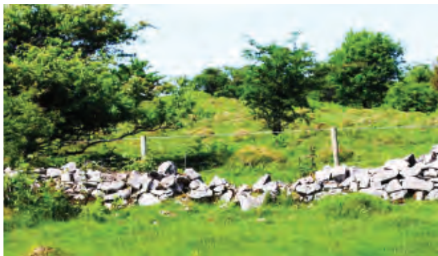
A slumped wall
