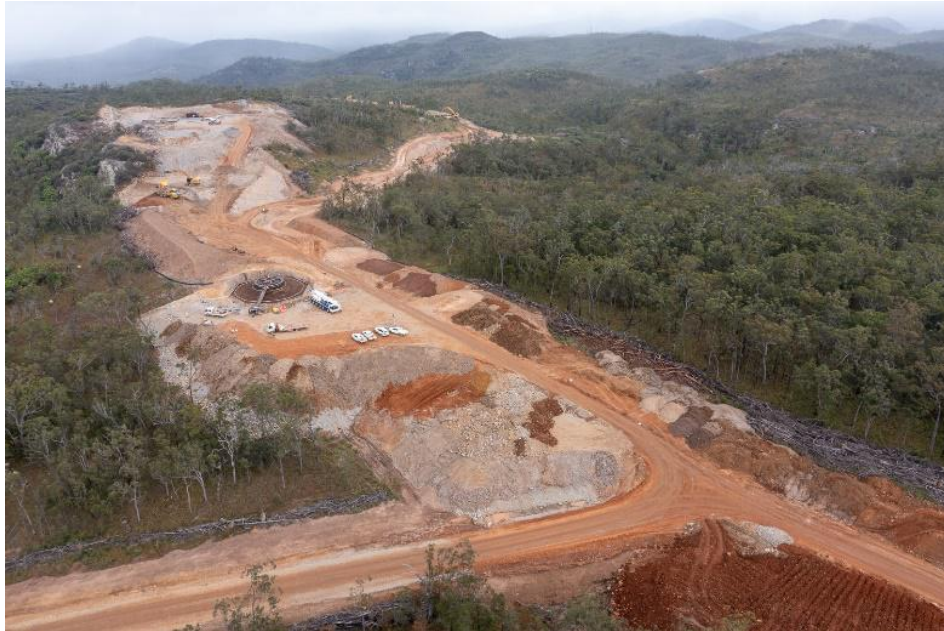
Kaban Windfarm construction
