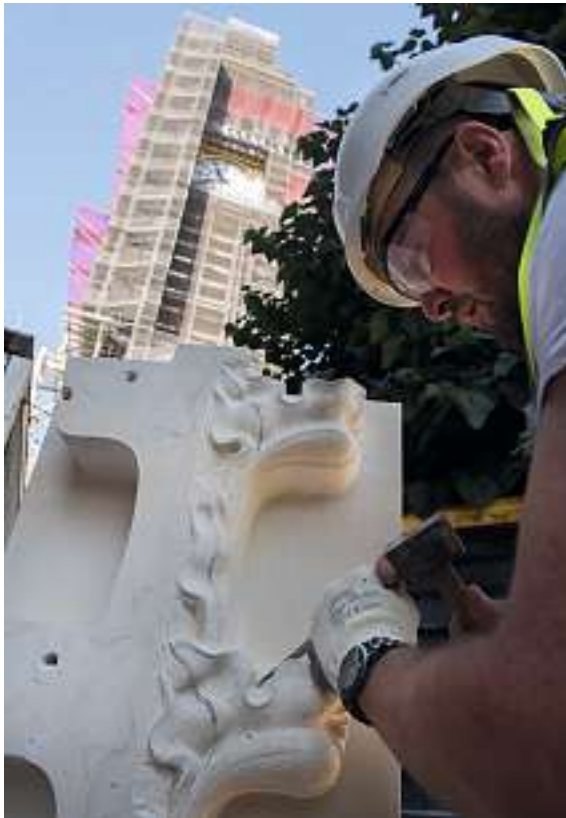
Left Carving Cadeby magnesian limestone, chosen to closely match the original Anston stone. Around 1,000 pieces have been replaced.
