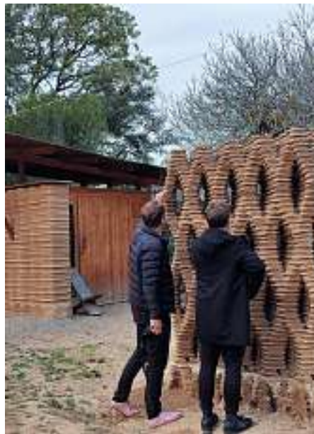
Below The weaving of the earth walls is customised to materials and climate, ensuring structural integrity while providing a porosity absent in most earth construction.
