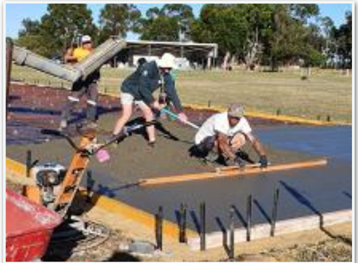
Pouring the concrete runway
