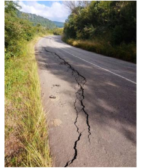
Cracks and damage to the Pilgrim's Rest main road (R533) on 22 April 2025, caused by destabilisation linked to illegal mining activity adjacent to the road.
